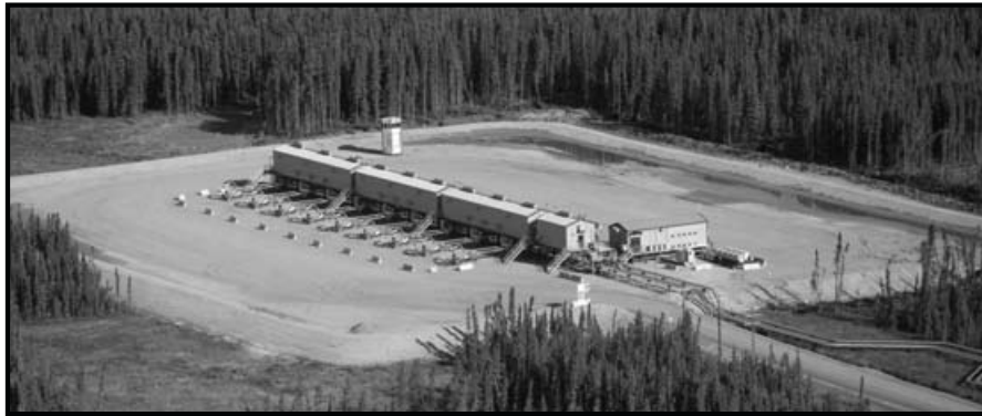
Figure 4 SAGD Well Pad and Central Facility
